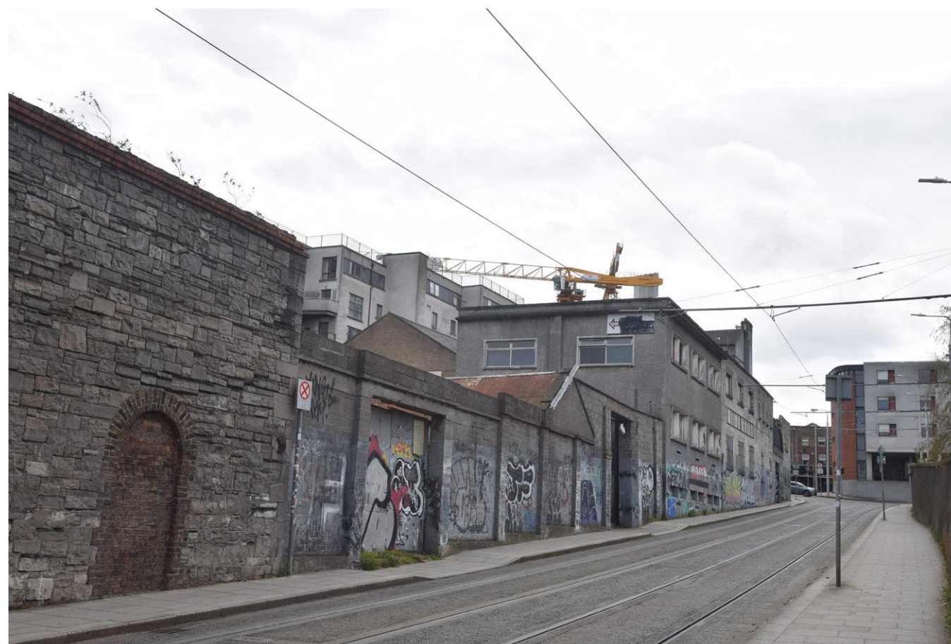
EXISTING VIEW FROM STEEVEN'S LANE (LOOKING SOUTH)
